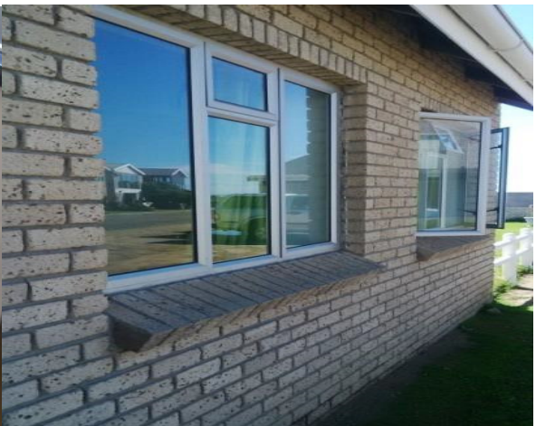
Old wood window frames replaced with aluminium frames at Stywelyne
