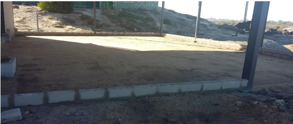
Extension of recycle plant Velldrif
