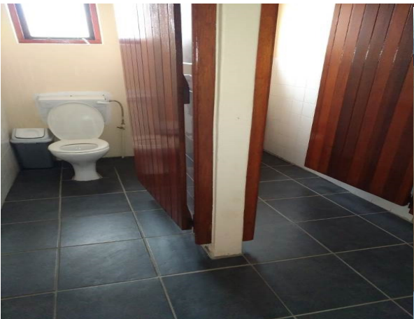
Upgraded ablution facility at DKB
